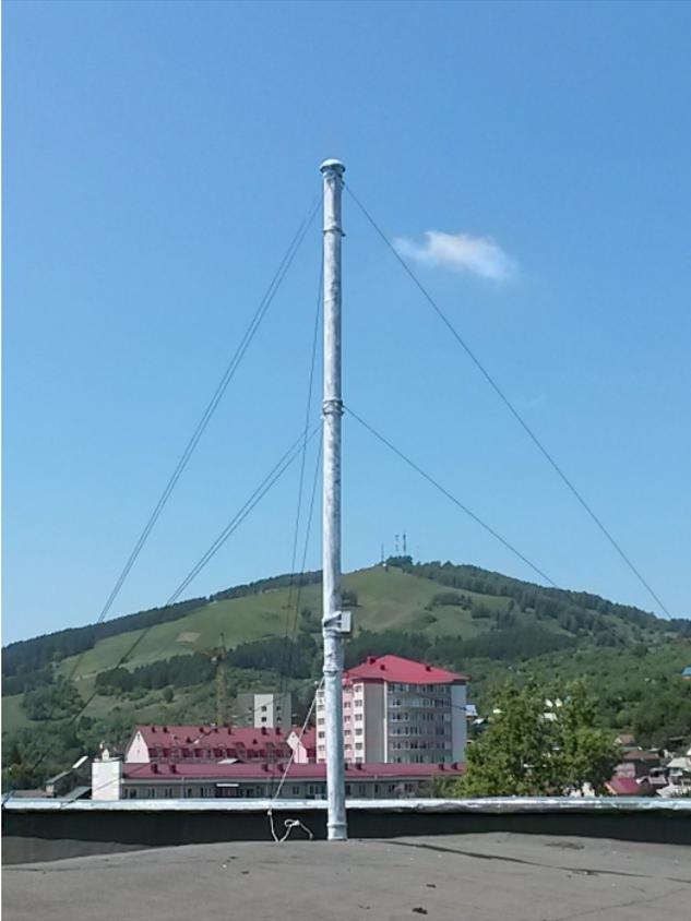
**Figure 1.** Antenna system of the WWLLN station Togagasu.
